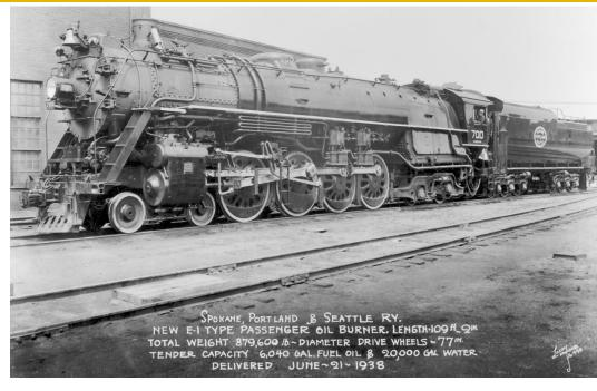
The 700 is A 4-8-4 (Northern) design, built by Baldwin to sister railroad (and one of the SP&S owners) Northern Pacific specifications. The engine started on the production line as a Northern Pacific A-3 with the main difference and change being the conversion to oil for fuel instead of coal. These became class E-1 locomotives on the SP&S.
